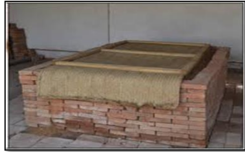
Ishusho ya 69: Ahantu hakonjesha umusaruro w'imbutu hubatswe ku murima hadakoresha ingufu z'amashanyarazi 24
